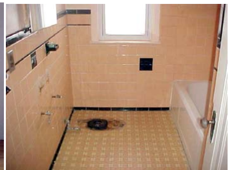
Bathroom, new sanitary units will be fitted
